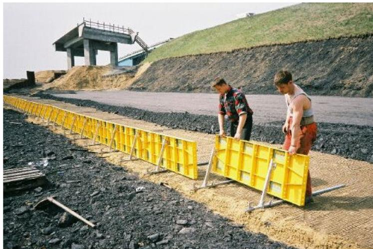
Photo 1. Installation of subsequent layer of reinforcement using the climbing shuttering by INORA<sup>®</sup> Ltd.
